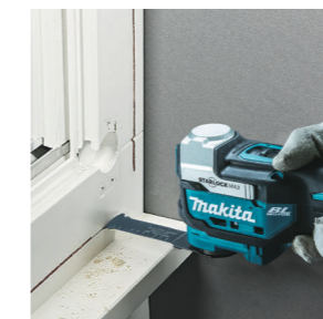
Removal of window frame
